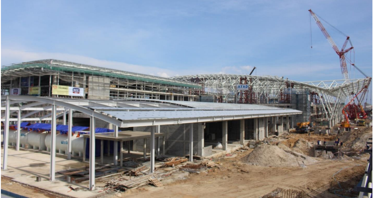
Picture: Terminal 2, Da Nang International Airport is on construction
