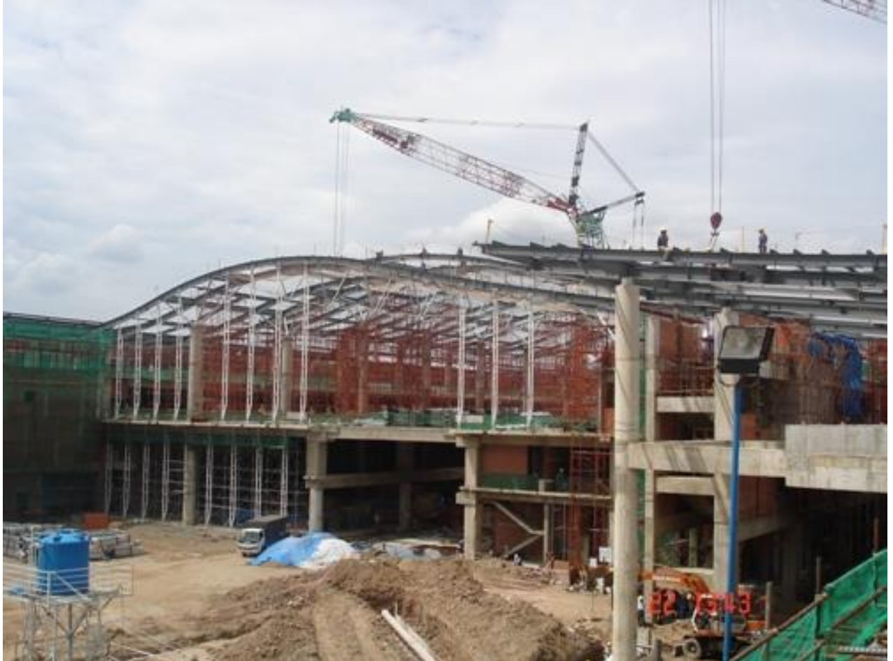
Tan Son Nhat Airport under construction
