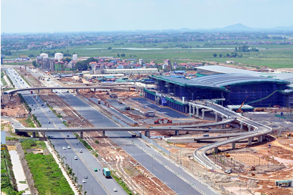
Noibai International Airport under construction
